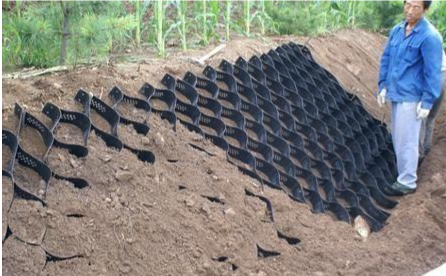
Figure 8: Geotextile matrix used for slope stabilisation (Source: https://www.okorder.com/p/hdpe-geocell-with-certificate-for-road-construction_1031785.html )
