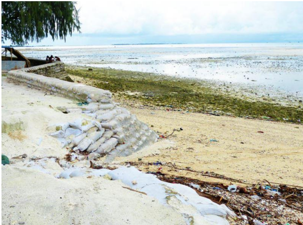
Figure 6: A hard seawall in Tarawa, Kiribati (SPREP, 2015)
