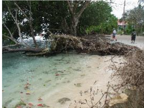
Erosion and undercutting of vegetation between Taro wharf and fisheries centre, threatening houses and infrastructure.
